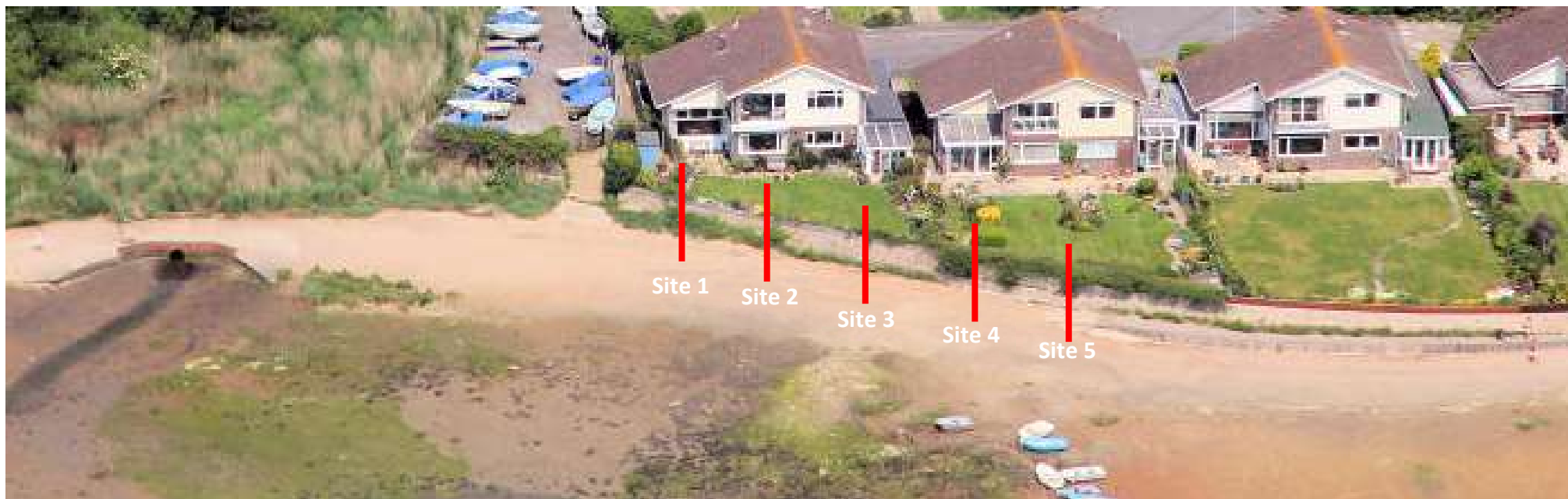
Location of measured data points (site locations approximate), along Maisemore Gardens frontage. Data provided by Maisemore Gardens residents. Photography ( www.maisemoregardens.co.uk )
