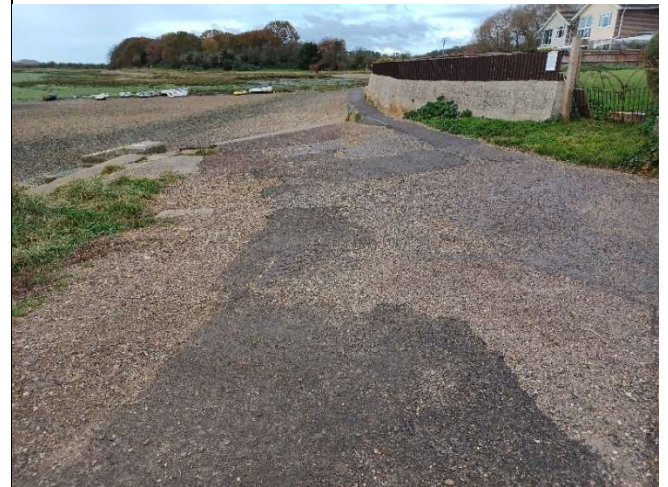
Plate 5: western end of seawall – ramp meets the foreshore – historical repair now undermined
