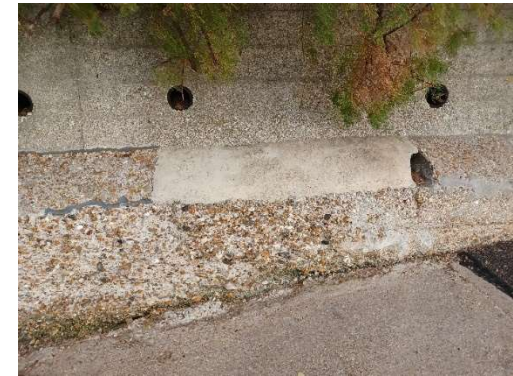
Plate 2: Face of seawall with drainage channels
