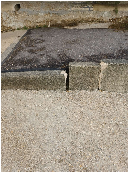
Plate 3: damaged capping stones at edge of footpath
