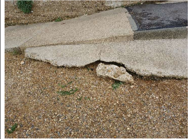
Plate 5: western end of seawall – ramp meets the foreshore – historical repair now undermined
