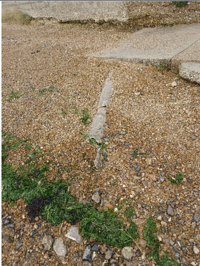
Plate 3: damaged capping stones at edge of footpath
